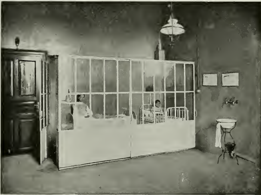
Steam-room. In the adjacent room there is a copper boiler, heated by gas and discharging steam through a copper pipe in the wall into the steam-room; an automatic regulator keeps the water at a constant level. Maximum capacity, six children. Children's Clinic, Gratz, Prof. Pfandler.
